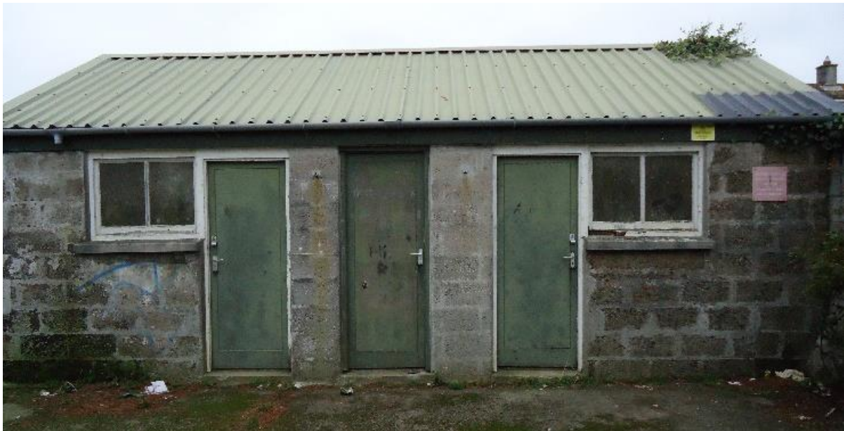
Original building that has been removed.
